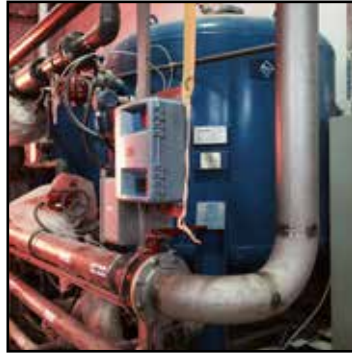
Photo: Napier Reid Filter Vessel
